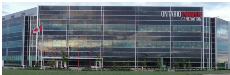
Figure 4-4 Darlington Energy Complex
