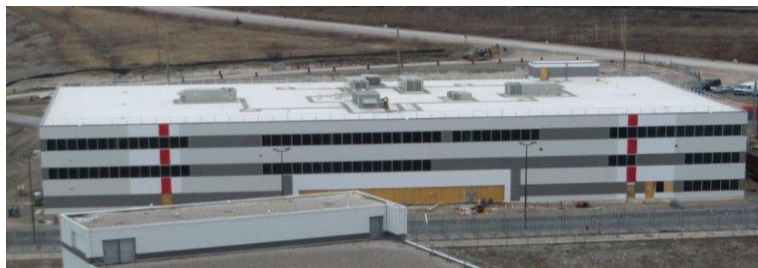
Figure 4-6 Refurbishment Project Office
