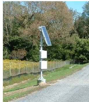
Figure 3-24 Gamma monitor located at Darlington site boundary
