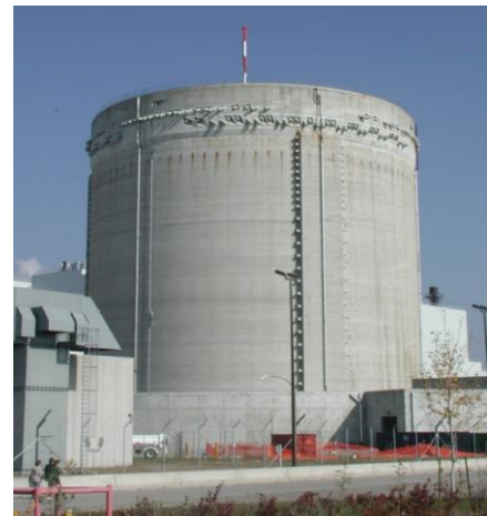
Figure 3-7 Darlington Vacuum Building
