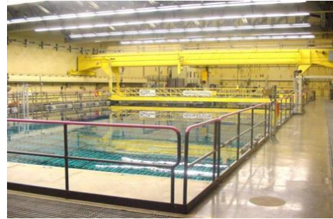
Figure 3-28 Darlington Irradiated Fuel Bay
