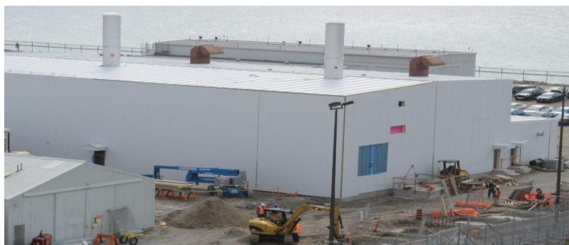
Figure 4-8 Auxiliary Heating Steam Facility
