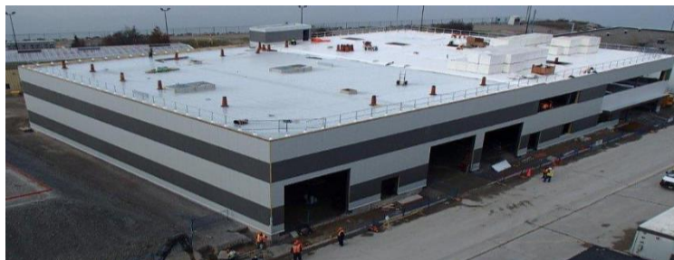
Figure 4-5 Re-tube and Feeder Replacement Island Support Annex
